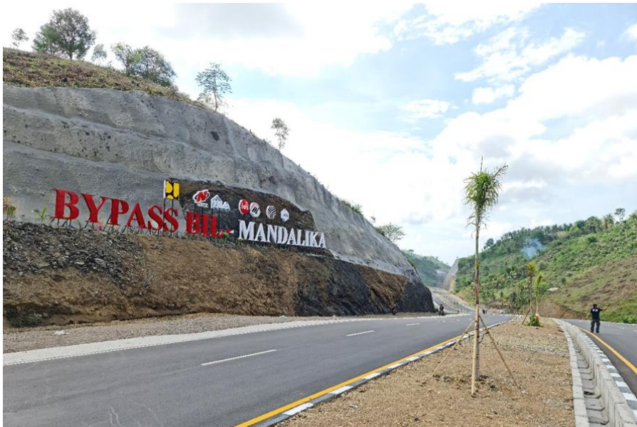
Gambar 4.8 Jalan Bypass Bandara Internasional Lombok - Mandalika
